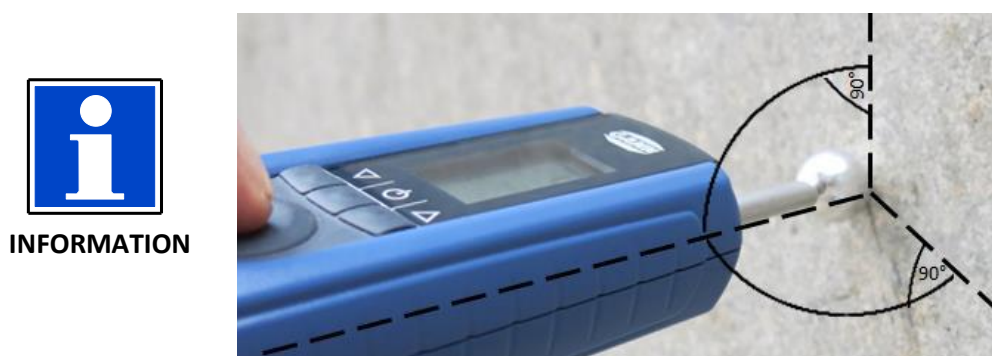
Figure 9-3: Measuring as vertically as possible to the measurement area
