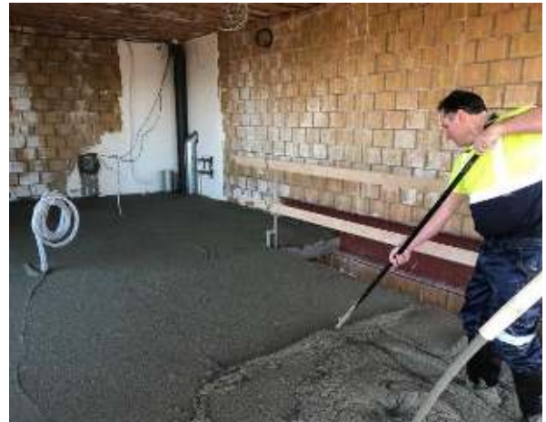
Figure 3: baseTherm® pumping and levelling
