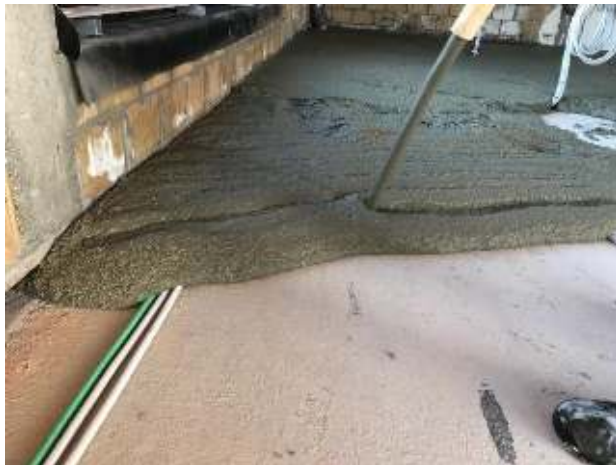
Figure 3: baseTherm® pumping and levelling
