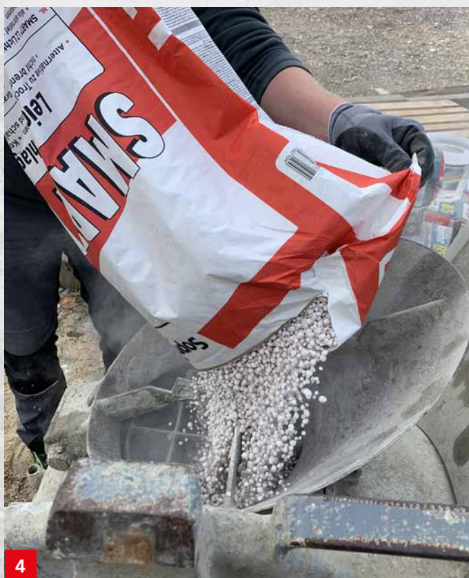
4 For larger areas, the use of a screed pump is recommended. First add Sopro SMART® LZ lightweight aggregate, then Sopro Rapidur® B5 or SoproTherm® SE-Z, and finally the required amount of water to the screed pump.
