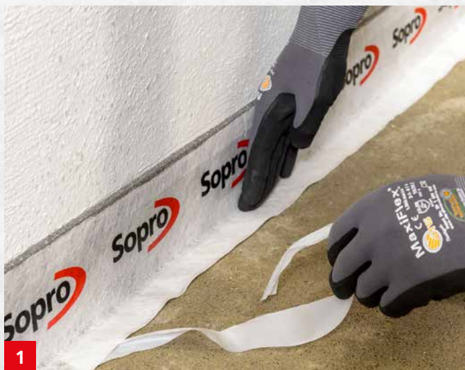
1 Fix perimeter insulation strip.
