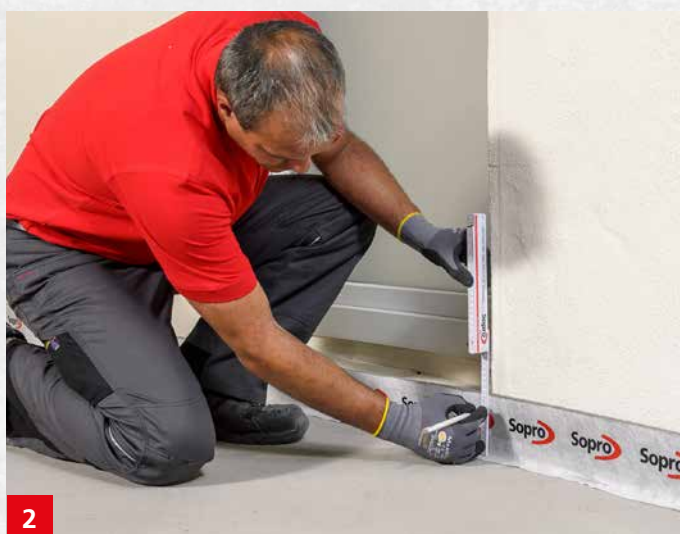
2 Mark datum line and reference points in accordance with required installation levels: Sopro SMART® lightweight levelling layer (> 20 mm 1)), Sopro VS 582 self-levelling filler (> 10 mm), adhesive coat and ceramic thickness.
