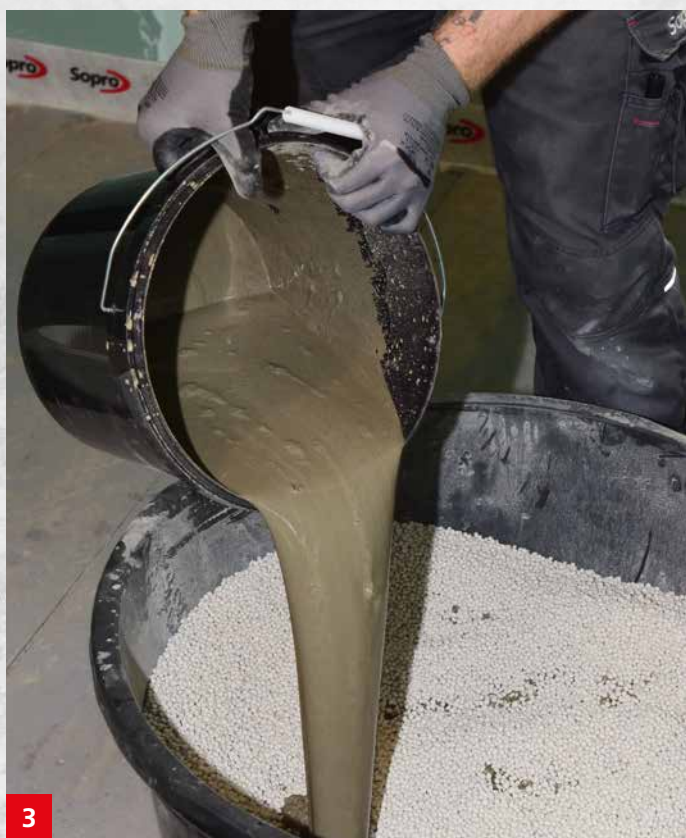
3 Mix 18 kg Sopro LZ 987 SMART® lightweight aggregate with approx. 12.5 kg Sopro Rapidur® B5 rapid-set screed binder and approx. 6.5–7.5 ltr water. Use of forced-action mixer is recommended for larger areas.
