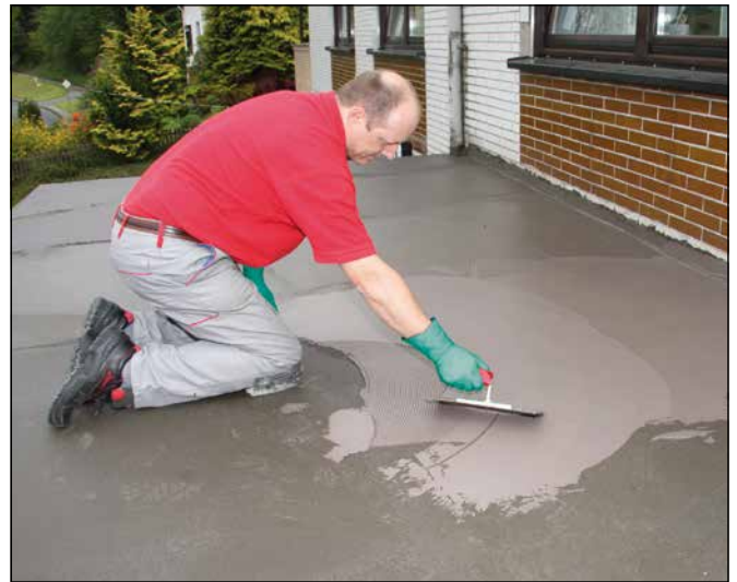
14 Apply second coat when first waterproofing coat has fully dried (after only 2 hours) ...
