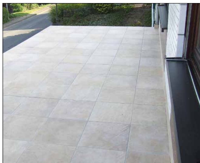
24 Fresh balcony tiling installed using Sopro system components.
