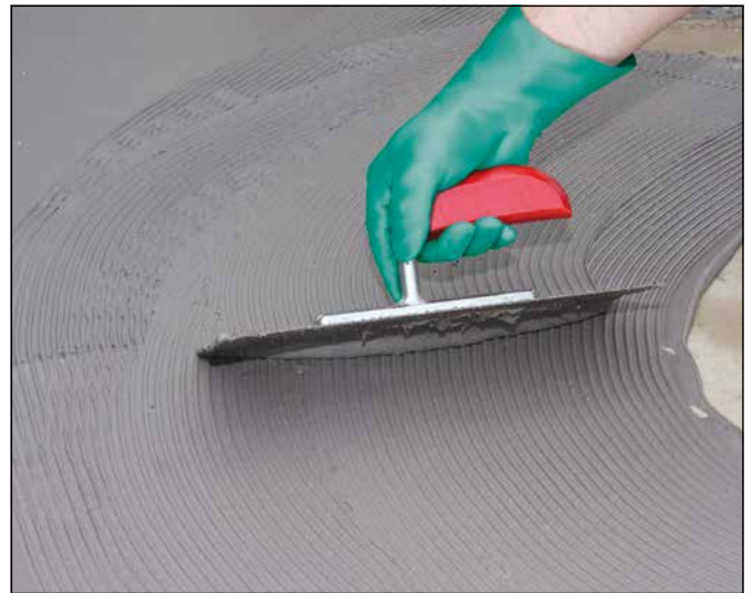
10 Apply Sopro TDS 823 to dampened or primed substrate using 4 mm notched spatula.
