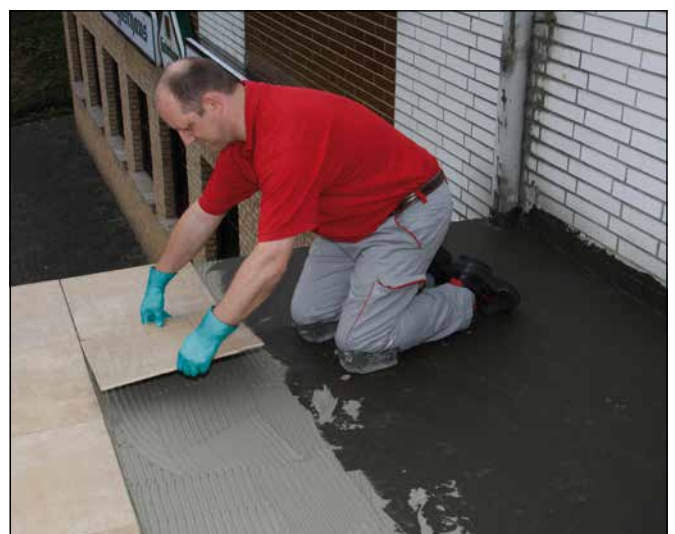
18 Place tiles in freshly placed adhesive bed and align.
