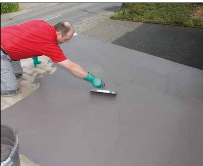
11 Smooth down Sopro TDS 823 with finishing trowel.
