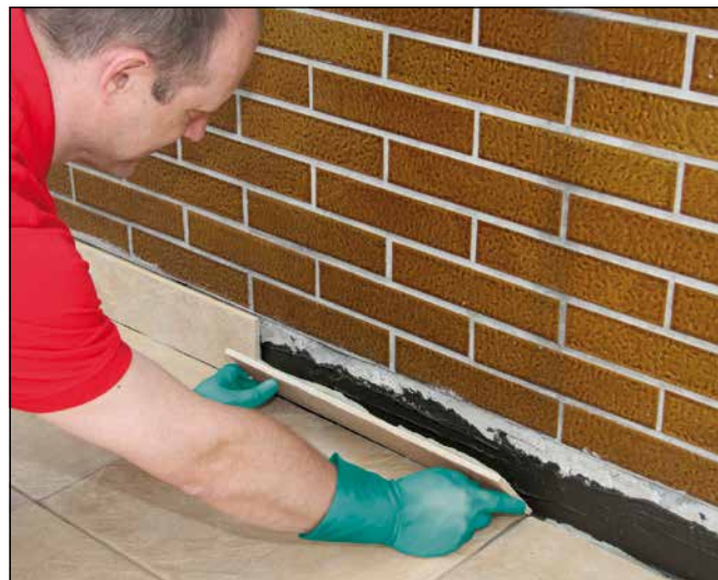
20 ... and place tiles in position.
