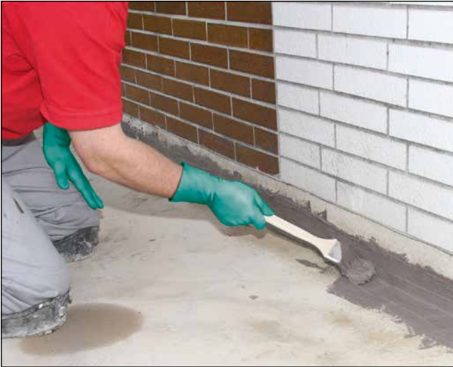
7 Coat area of wall junctions with Sopro TDS 823 to allow ...
