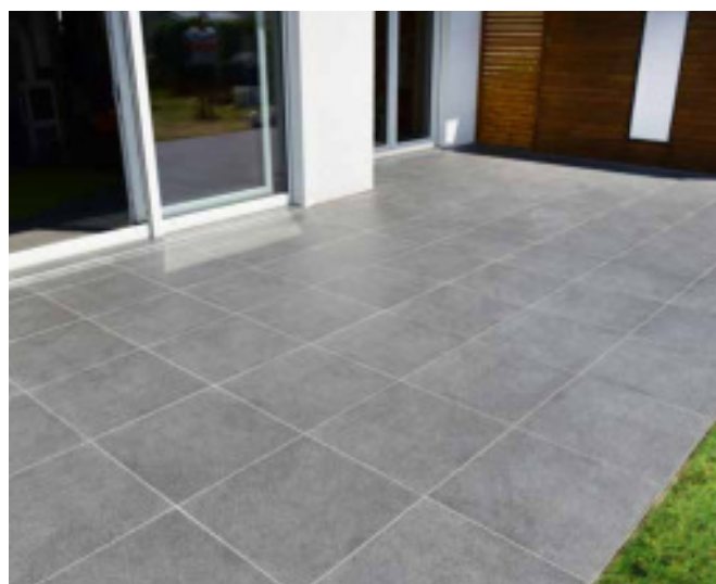
18 Grouted surface is walkable after 24 hours.
