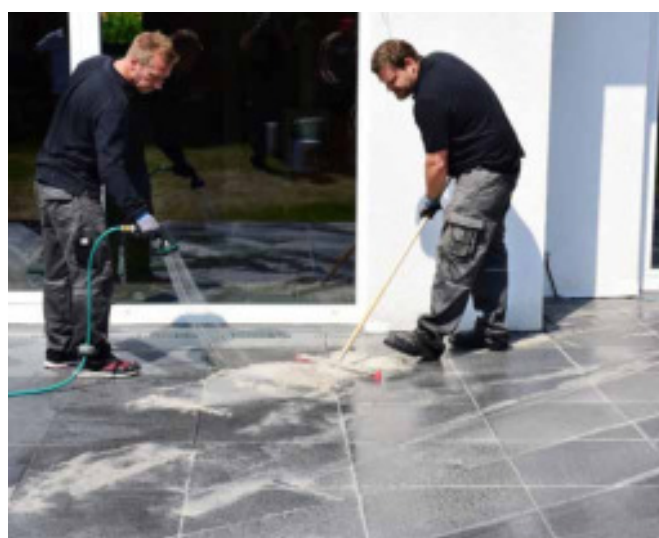
12 Dampen material with water jet to achieve smooth, workable consistency...
