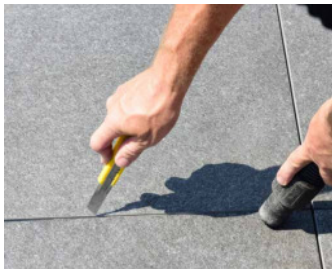
8 Thoroughly clean joints and remove all residue.
