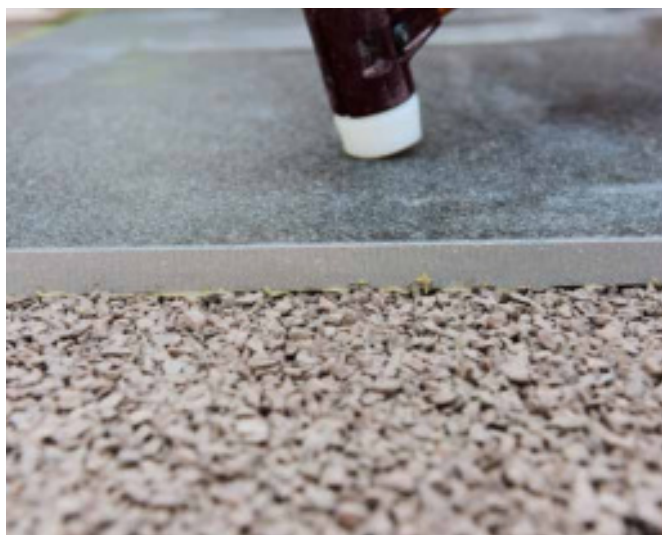
7 Position tiles and tap into place.
