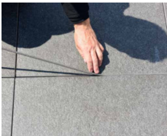
9 Install back-up strip in specified movement joints to prevent three-side adhesion.
