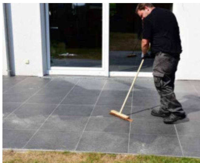
16 ... and, where necessary, sweep away mortar residue.
