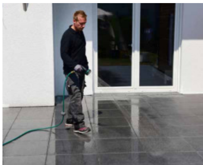
10 Thoroughly pre-wet surface prior to grouting and keep in damp condition.
